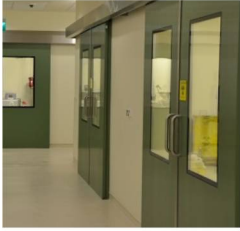
SIO LEAD LINED DOOR
